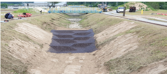
Fig. 1. Fishway installed using biopolymer.
